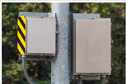
Control enclosures mounted to each of the 30 gantry poles include all low voltage, high voltage wiring and fiber connections.
