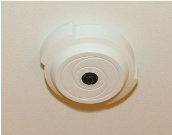
Cal Coast Telecom installed Pelco 360-Degree cameras, providing the new digital CCTV system total situational awareness and video motion detection.
