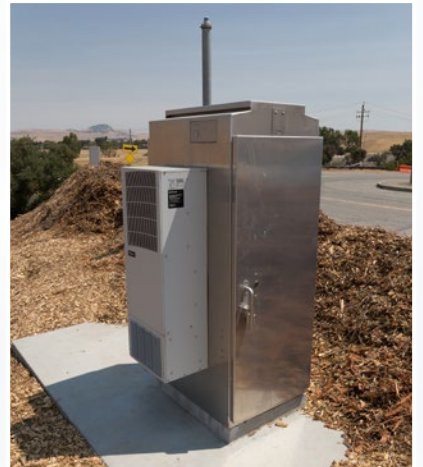
All low voltage power and fiber from the control cabinets at the gantry poles were then routed to 39 enclosures installed on the side of the freeway. These enclosures are then connected to the central control center.
