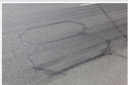
Rosendin Electric also installed induction lane loops in the pavement to count cars as they pass, helping to judge how heavy traffic is.
