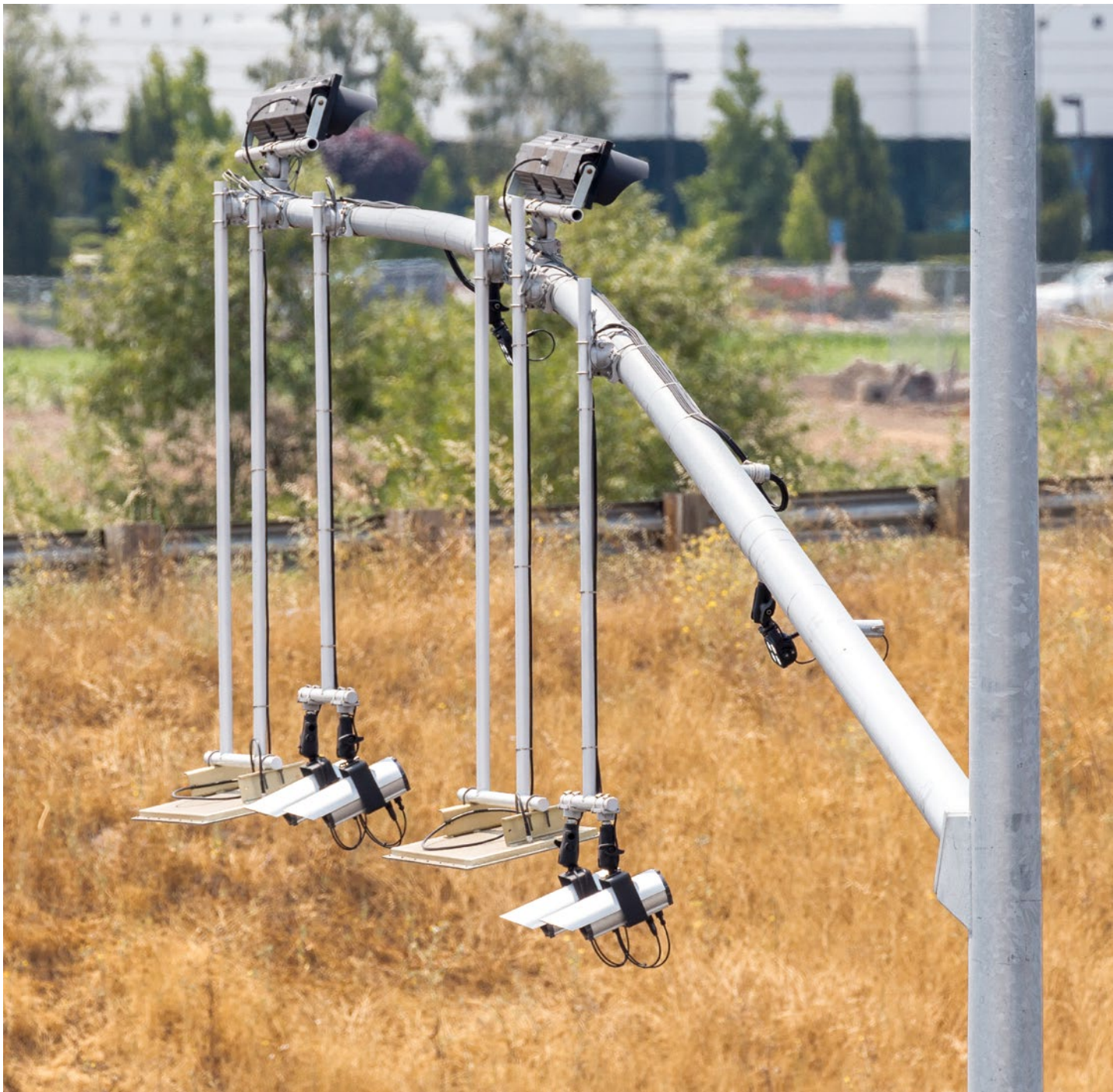
Rosendin Electric installed many devices to help monitor traffic, including CCTV, overview cameras, and LED lights across 30 gantry poles placed along the route.
