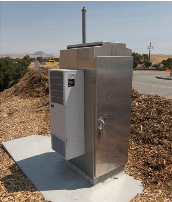
Rosendin installed 39 enclosures on the side of the freeway which route the gantry pole wiring to the central control center.
