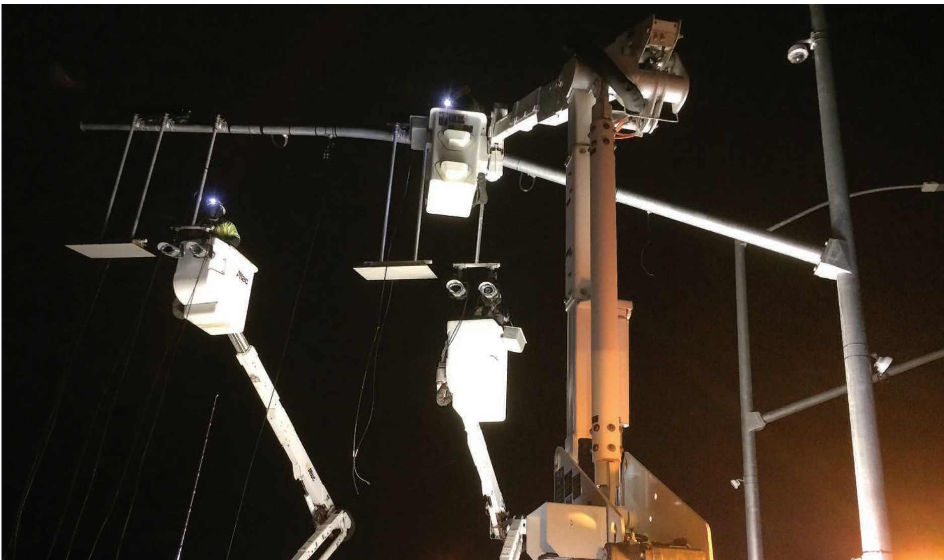
Rosendin Electric wires low voltage power in the new I-580 express lanes.
