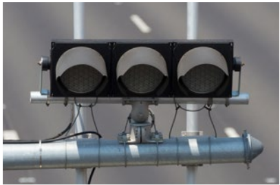
Beacon lights are triggered by the antenna card reader and show the presence and setting of FasTrak toll tags.
