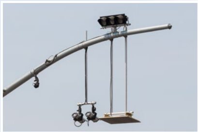
Many of the devices installed by Rosendin Electric on the 30 gantry poles within the toll lanes help to monitor traffic flow. These devices include an antenna card reader, a violation enforcement camera, beacon lights, a CCTV camera, and LED lights.
