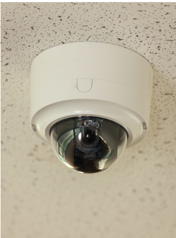
The Pelco Pan-Tilt-Zoom (PTZ) cameras installed are capable of remote directional and zoom control.
