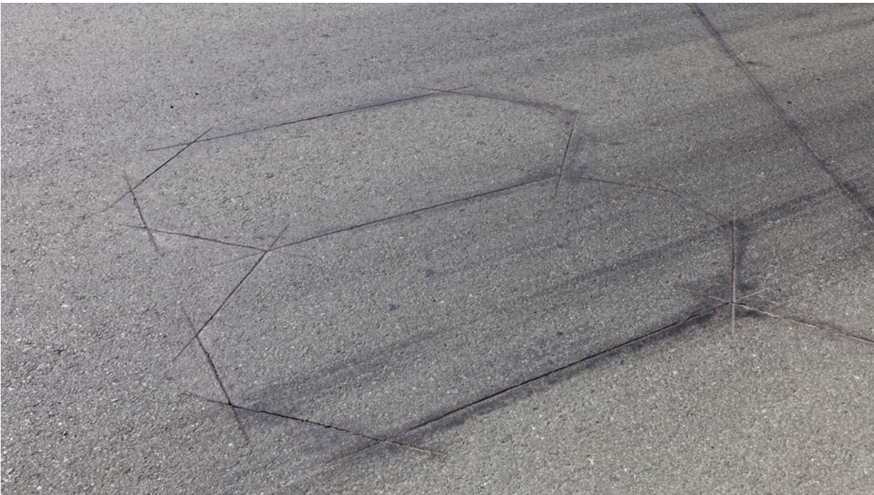
Induction Lane Loops and Magnetometers were installed along the 14 miles Express Lane for real time monitoring of the flow of traffic.
