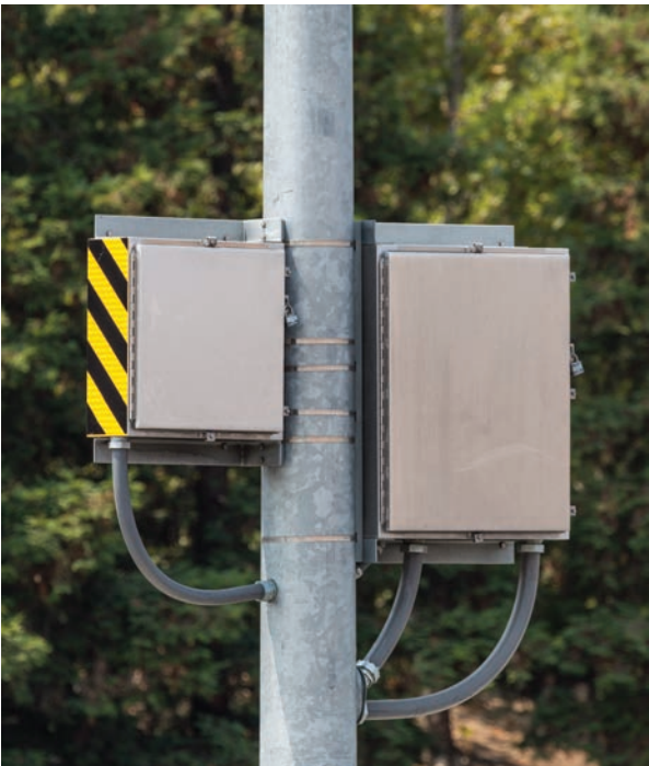
Control enclosures mounted to each of the 30 gantry poles includes all low voltage, high voltage wiring and fiber connections.
