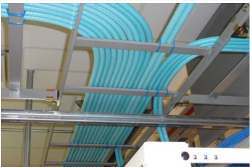
Fiber optic cabling
