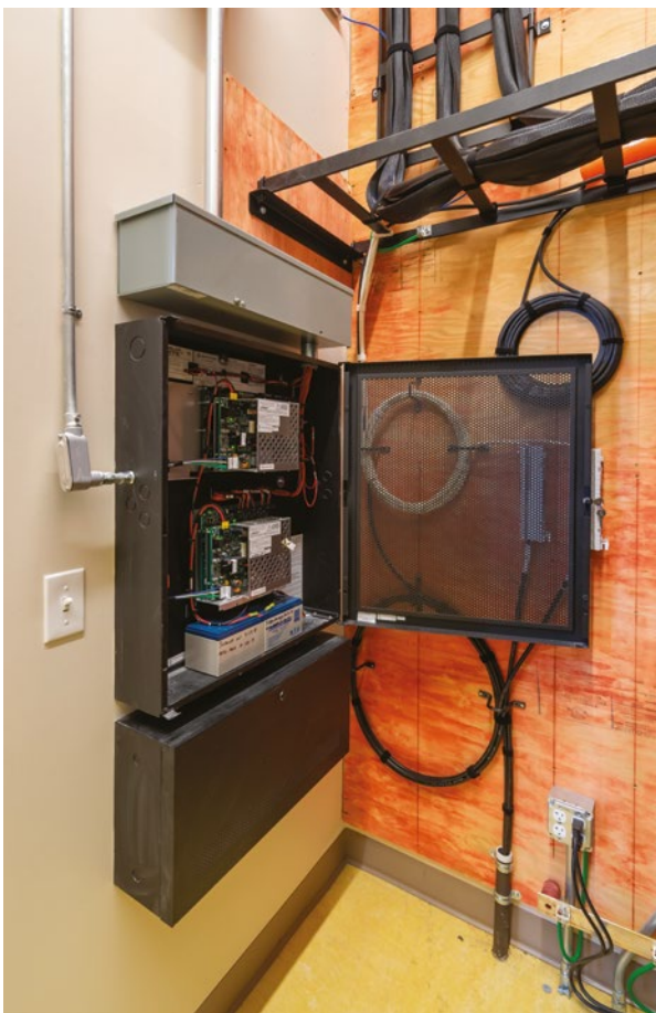
Intrepid's work included building the main fire alarm panel and sub panels.
