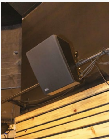
PCD installed Meyer Sound Laboratories UPQ-2P coverage loudspeakers.
