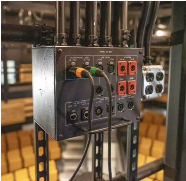
PCD installed patch panels throughout the theatres to reinforce the new sound system.
