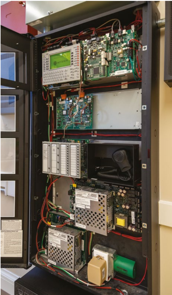
Intrepid chose a Honeywell Notifier 3030 (NFS2-3030) panel for the new voice evacuation fire alarm system.
