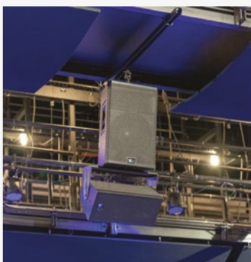
PCD installed speakers in clusters at the front of the stage, along with overhead speakers.
