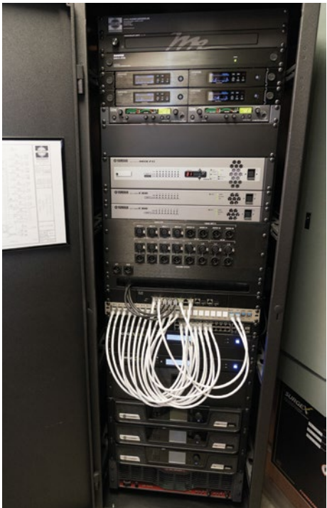
The adjoining control room holds JBL and Yamaha audio reinforcement systems; power conditioners are used to clean up excess noise.
