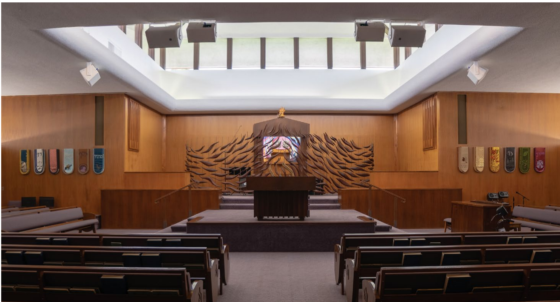
Six speakers and two subwoofers were installed in the sanctuary providing optimal audio coverage of the new sound system.
