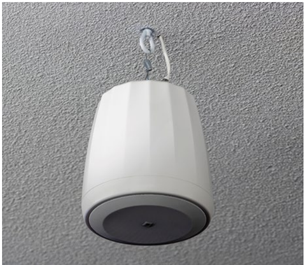
Twelve JBL pendant speakers were installed on the ceiling in the social hall.
