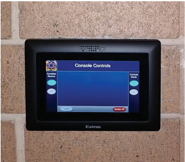
A Extron touch-screen provides easy-to-use control over the sound system.
