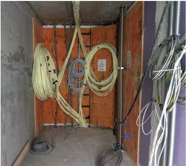
McMillan Data Communications installed a total of 30 IDF rooms and brought the connection from the main point of entry (MPOE) within the building.
