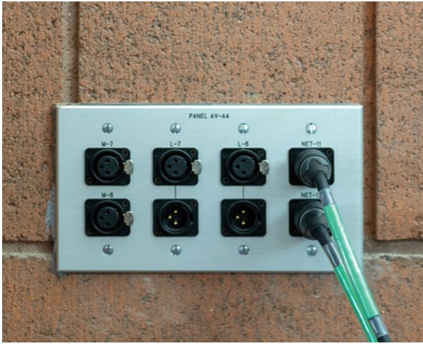
An installed AV panel connects the sanctuary to the control room.
