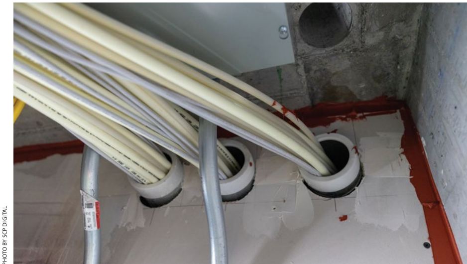
McMillan Data Communications is also installing two microducts, one for Comcast and one for AT&T. The microducts are small plastic conduits to install fiber optic cable through the ceilings and walls after construction.
