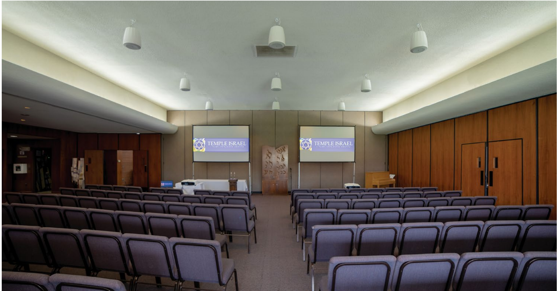
Twelve JBL pendant speakers were installed on the ceiling in the social hall.
