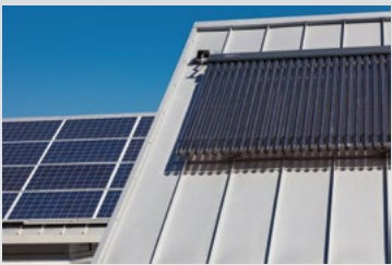
Roof Monitors With Solar Thermal Glycol Panels
