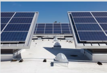
Roof Monitors With PV Panels
