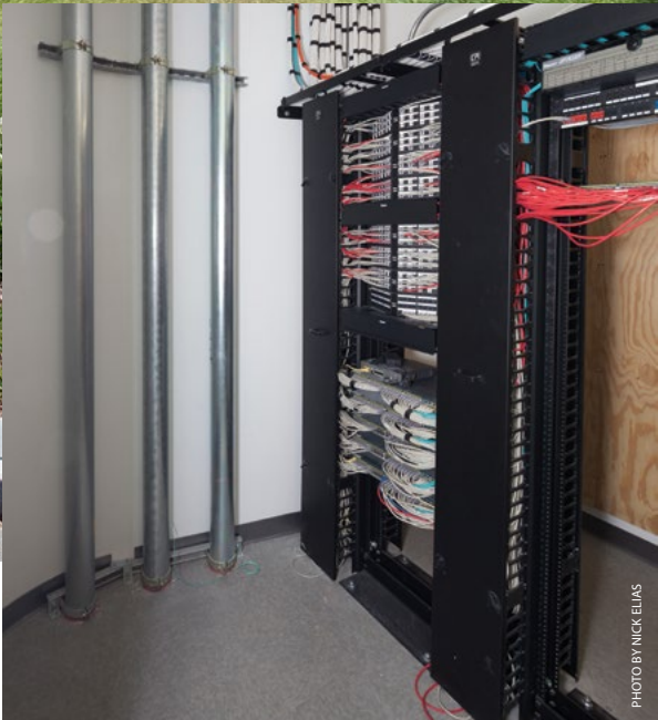
The structured cabling system design enabled IDEX to terminate the 2nd floor cabling in the server room below.
