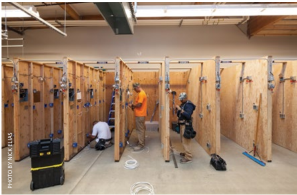
The ZNE building, with 14 training rooms, is used primarily to train both apprentice and journey level electricians. These students are being trained at workstations in the Dick Nordeen Tool Lab.
