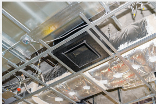
Walker Telecomm has roughed in the structured cabling for the AV, including back boxes for subwoofers.
