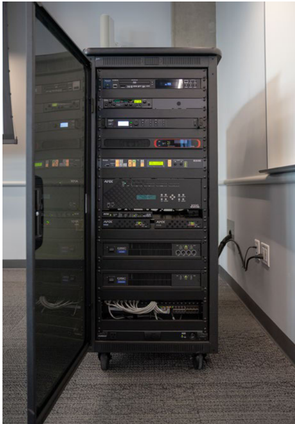
ICS custom built portable racks which include an assisted listening component.
