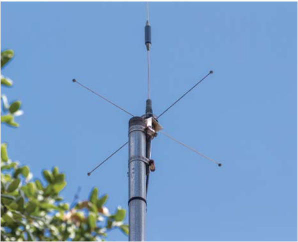
Intrepid Electronic Systems installed exterior RF Antennas to monitor building and maintenance records, and report the current status of the system and its individual devices via a mesh network.
