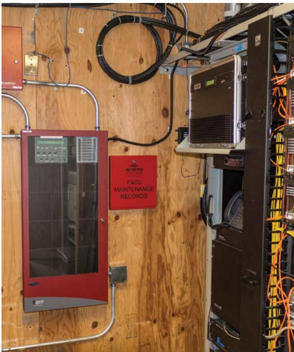
Intrepid Electronic Systems installed the AES-IntelliNet Fire Alarm reporting system, which via the fire alarm panel monitors and reports the status of all the fire alarm devices via a RF mesh network.
