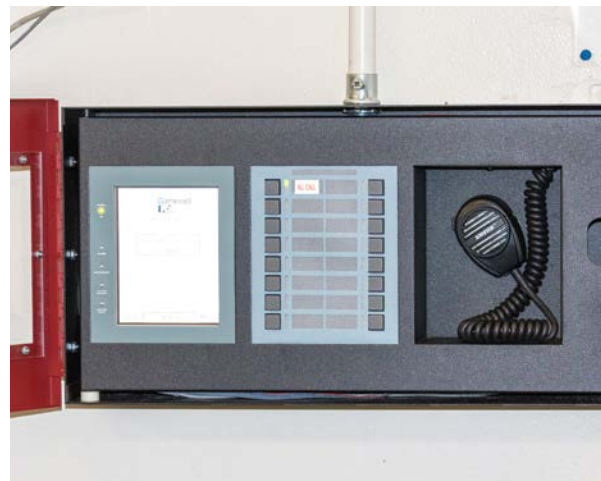
Intrepid Electronic Systems installed network graphic annunciators which are used to convey to the students the steps needed to be taken during an emergency.
