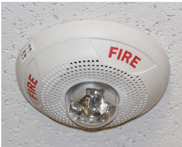
Intrepid Electronic Systems wired each room in the schools with a speaker strobe notification system which alerts students of an emergency and provides directions on how to proceed.
