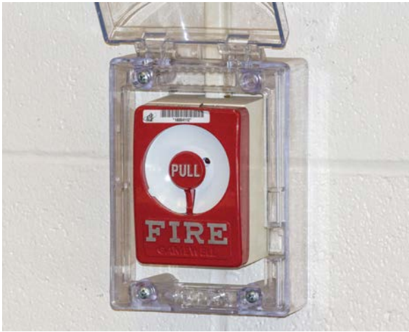
A pull station fire alarm is installed in public areas, such as auditorium or gymnasium, not in a classroom. This allows for manual activation in a populated space.
