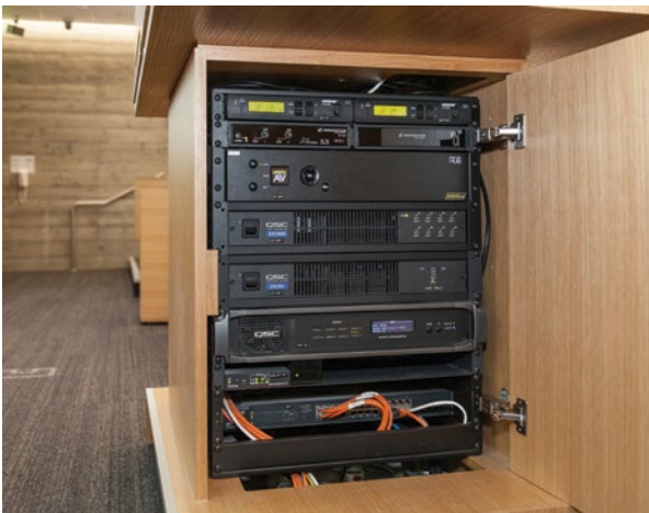
ICS installed the audio-visual processing equipment in a podium at the front of each tiered classroom.
