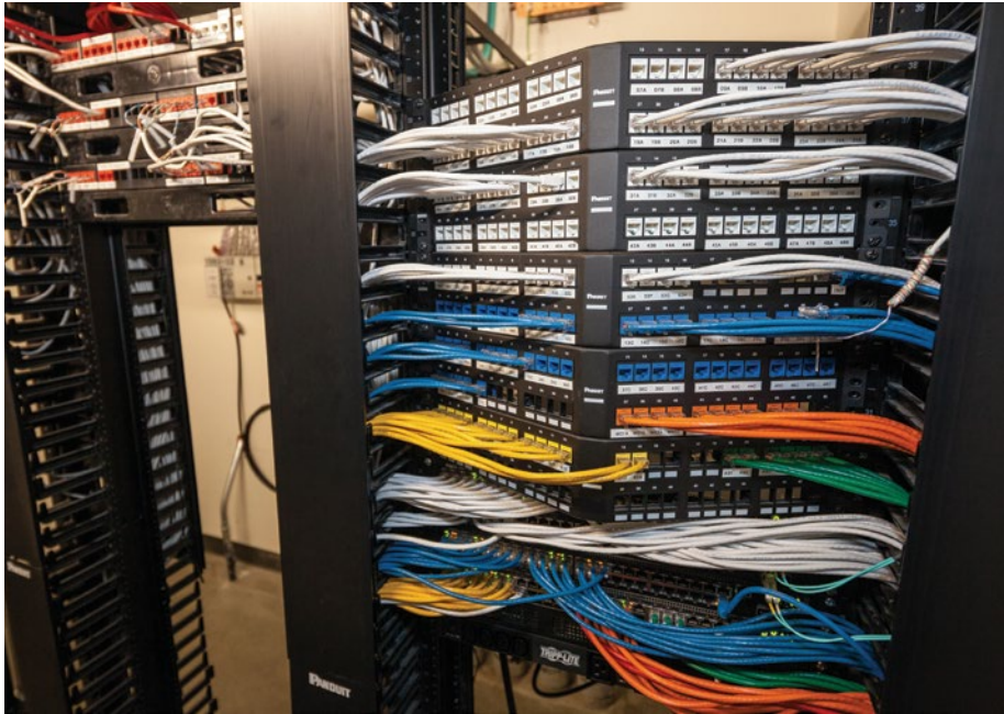
Paganini Communications wired a redundant fiber backbone system that runs between the five floors, and goes through the IDF rooms, which are stacked on each floor.
