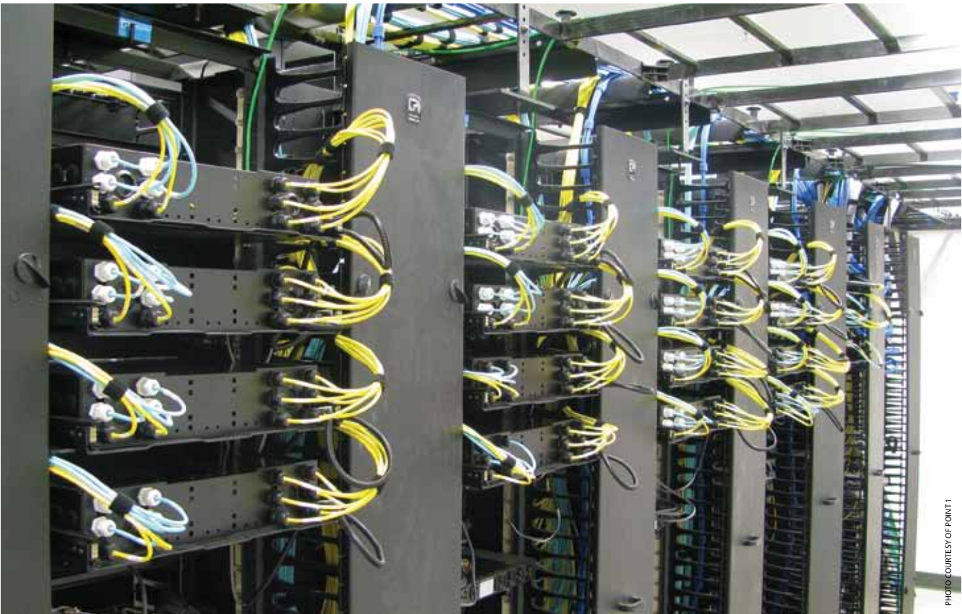
Wiring in the Telecommunications Equipment Room
