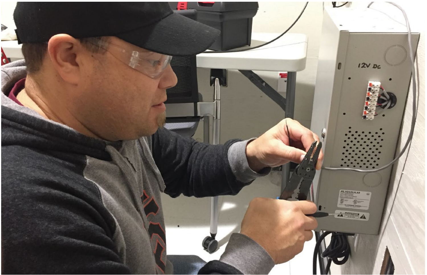
3rd Year apprentice Gerald Montgomery connects power for an analog camera.
