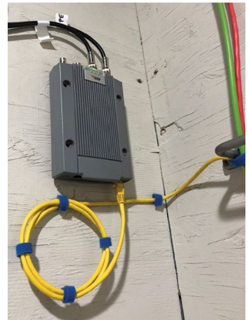
The JATC purchased the Axis Video Encoders to tie in the existing analog cameras for each of the eight labs.
