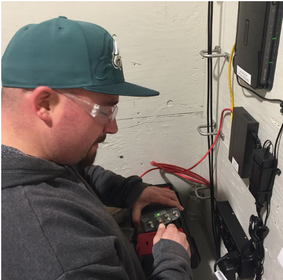
3rd Year apprentice Kyle Six connects an analog camera to the encoder.
