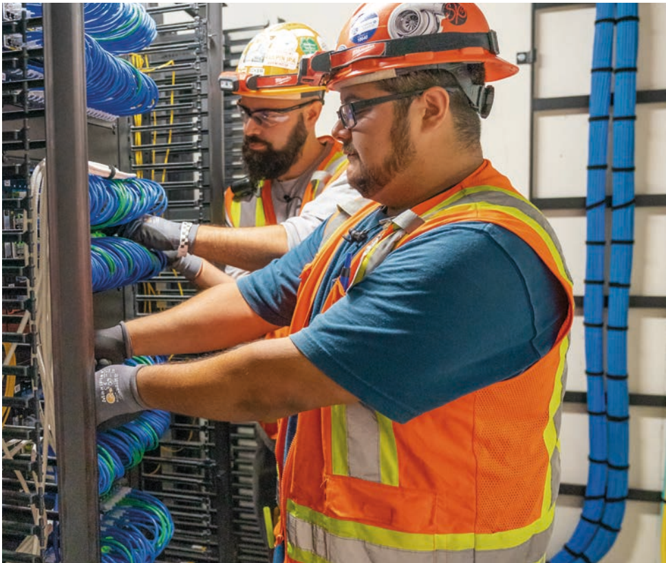
Kris Basurto and Ray Malaspina of Decker Electric place patch cords from patch panels to the switches.
